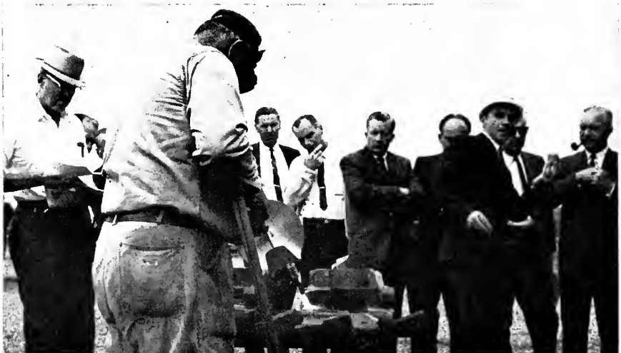
Members of Committee 22 inspect an operation in which worn retarder parts are repaired by first heating them to a temperature of 400 F and then applying a hardfacing powder.
